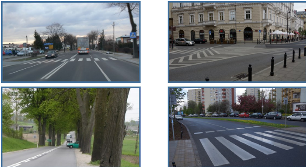
Fig. 3 Examples of road defects.
