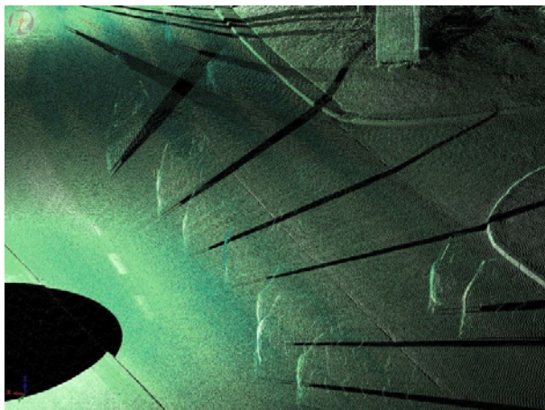
Fig. 3. Result of asphalt bus creek scanning.
