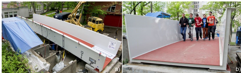
Fig. 8. GFRP footbridge constructed within Fobridge project.
