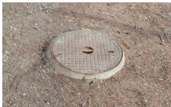
Figure 7-6: Shaft No. 3 on April 7 th , 2011. Possible uplift.
