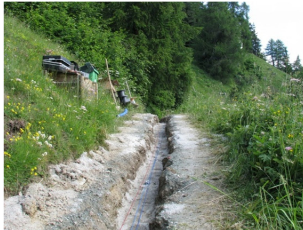
Figure 7-4: Trench with fiber optic sensor.
