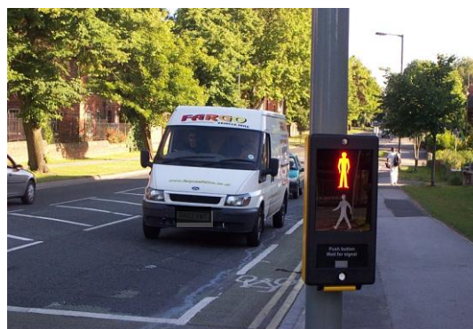
Figure 5.1: Pedestrian view of nearside signals, showing on-coming traffic in line of sight
