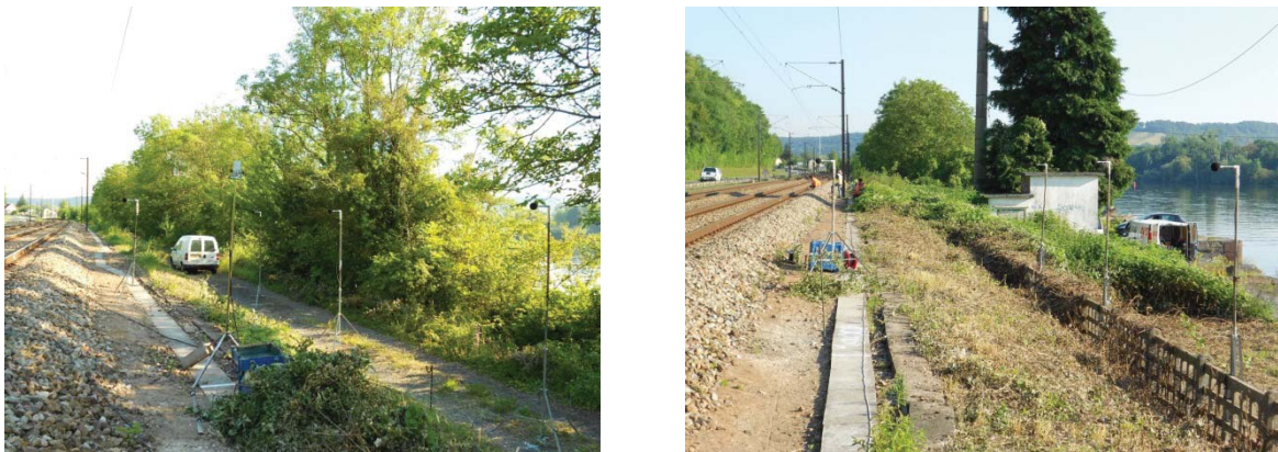
Fig. 80: Test track for field tests
