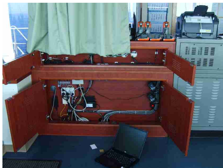
Backside of Bridge Computer office
