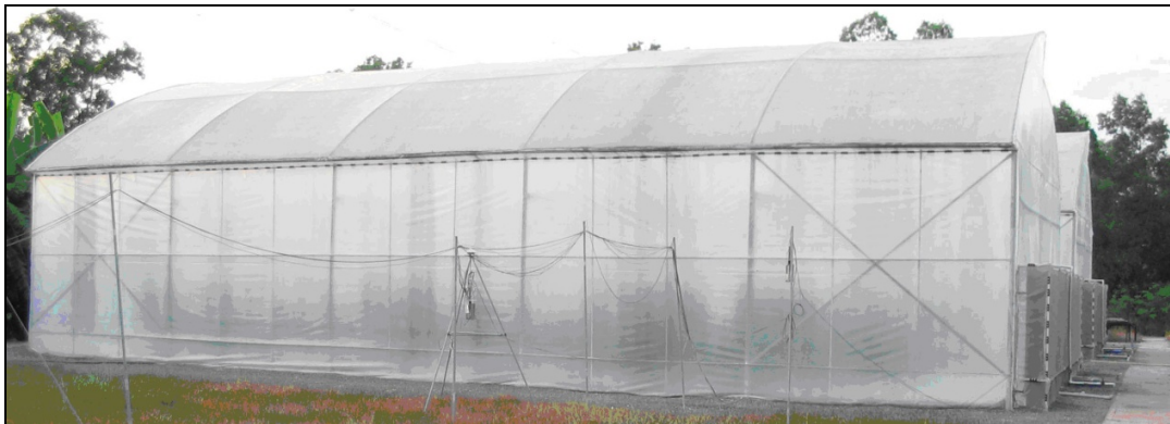
Figure 3.3.2. A photograph of the greenhouse equipped with a fan and pad cooling system (FAP) use for the experiments in Central Thailand. The cooling pad can be seen protruding behind the gable wall on the eastern end of the greenhouse.
